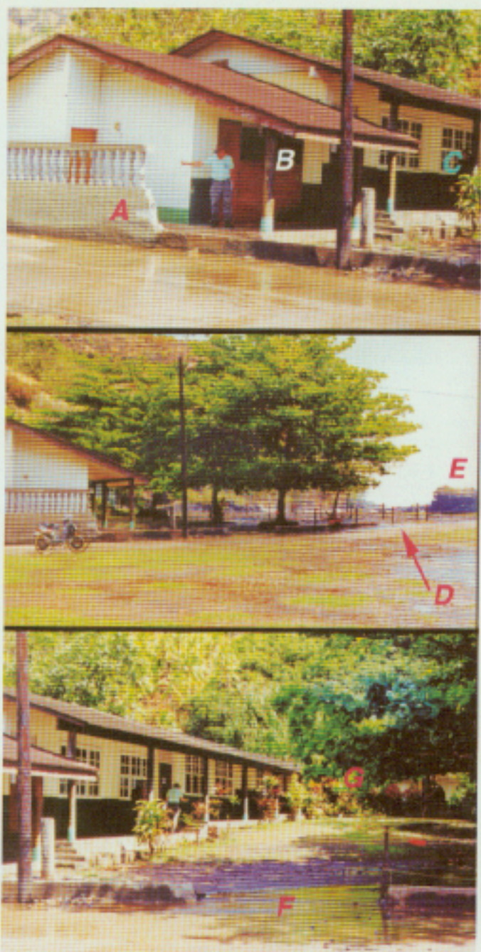
FIG. 3. – The damaged school at Omoa, photographed on 4 October 1999. Top (looking SSE) : The wall (A) has been totally destroyed around the playground. The principal's office and teachers' room (B) have been damaged and are now boarded up. Classrooms located at slightly higher elevations (C) were merely flooded. Center (looking SW) : The wall (A) used to extend all around the yard (to point D), and has been destroyed. Note the Motutapu promontory in the distance (E), which provided some protection to the southern part of the bay. Bottom (looking south) : (F) shows the location of the entrance gate through the wall. Note the slight incline to the south which lessened the impact of the waves on the more distant classrooms, and especially on the pre-school building (G; hidden beyond shrubbery).
