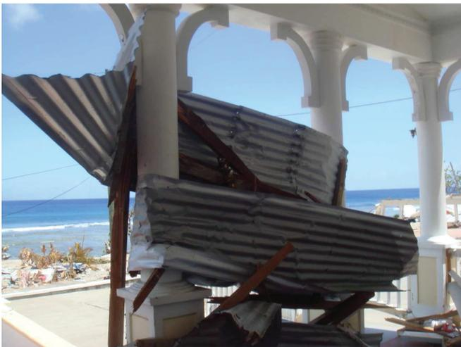
▲ **Figure 3.** Top: Devastation at Poloa, Tutuila, American Samoa, photographed six days after the event. The church building, behind which the highest run-up on the island, 17.6 m, was measured, is the only building left standing. Bottom: Close-up of a corrugated piece of roofing, wrapped around the pillars of the church porch.
